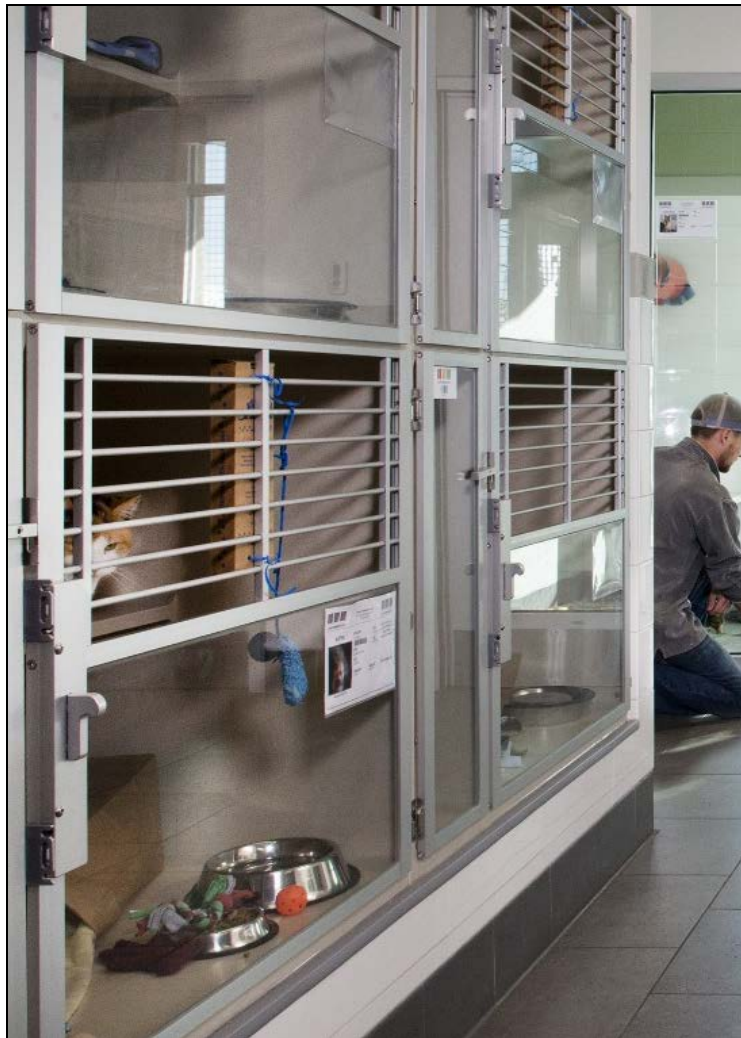
Cat housing with non-reflective interiors, horizontal bars, and resting benches Credit: Foto Imagery / Tim Murphy
